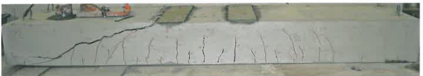
Fig. 3. Crack pattern after reaching shear force capacity in specimen V2Da of the Darmstadt tests [5]
