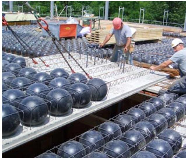
**Figure 1.2** Cobiax semi-precast slabs
