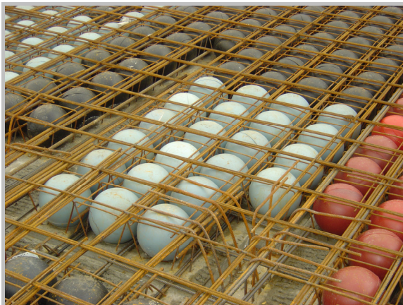
Figure 4 Cobix flat slab module
